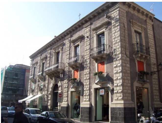
Fig. 9. Restoration site where the mortar was used – “Palazzotto Bis-cari”; Catania.
