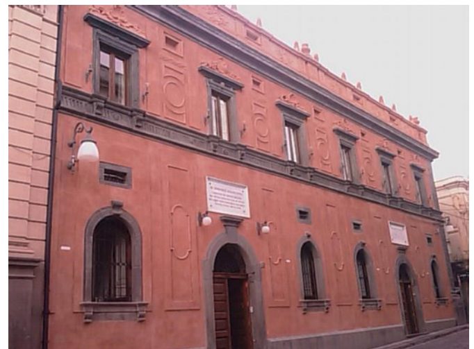
Fig. 10. Restoration site where the mortar was used - “Real Collegio Capizzi”, Bronte (CT).
