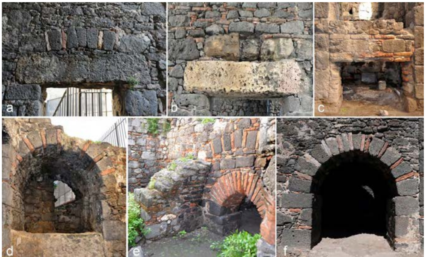
Fig. 13. Evidence of two lintels in the northern (a) and the southern wall (b) of room 1; (c) rectangular flue connecting the hypocaust of rooms 5 and 7; (d) arch in opus vittatum in room 3; (e) remains of a vault on the exterior wall of the niche 11; (f) arch in opus vittatum in room 12.
