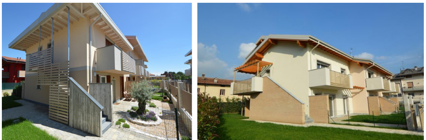
Fig. 2. On the left: Building A, built with a load-bearing structural system of cross laminated timber; on the right: Building B, built with a reinforced concrete load-bearing frame and brick walls.
