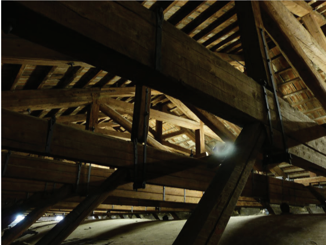
Figure 3. Roofing of St. Peter's Cathedral (shot by Stefano Lamborghini).
