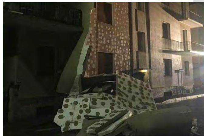
Figure 2. Shell thermal insulated envelope detachment due to the wind action (Brescia, 2016). In this case the insulating panels were fixed to the masonry support in a wrong way.
