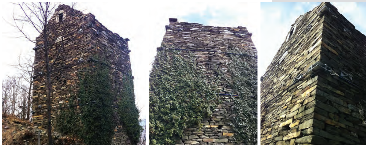
Figure 1a (left). The Lossetti Tower. Figure 1b (centre). One of the DSM walls of the tower: are clearly visible serious cracks. Figure 1c (right). Safety devices applied to the tower: steel ties and steel cables.
