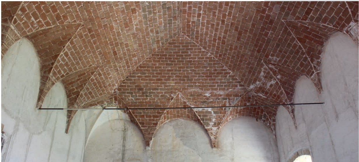
Figure 6. Realization of a tiled cloister vault with lunettes, taking place a collapsed stony one.
