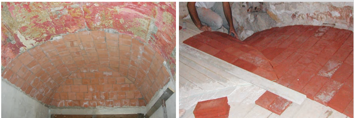
Figure 4, 5. Reconstruction of a partially broken down tiled vault. Philological reconstruction of a tiled barrel vault with lunettes.
