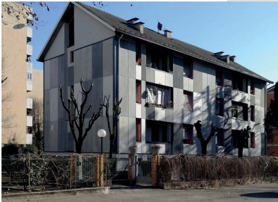
Figure 10. View of the South-West Façade after the EASEE panels installation.
