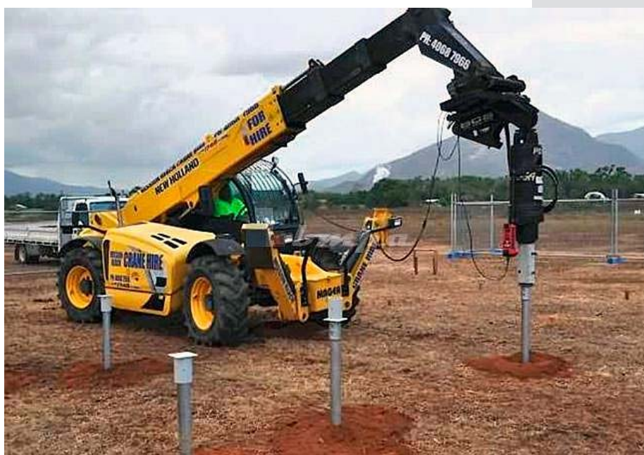
Figure 13. Installation of foundations on poles fixed by screwing ( https://goo.gl/images/mBTuSs ).
