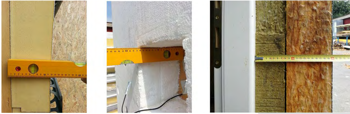
Figure 2. Picture of the three tested wall. Left: Polyurethane foam Isotec® Parete; Center: EPS panel; Right: double panel in high density rock wool.
