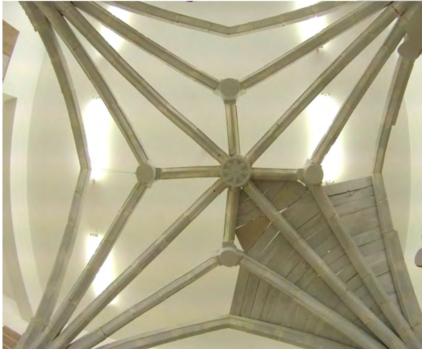
Figure 28. The structural rib system of the S. Maria della Catena church's vault, following dismantle phase. (©labstereounipa).
