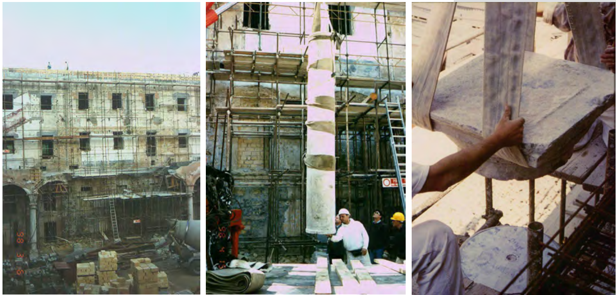
Figures 3, 4, 5. Construction of scaffolding; positioning of a new Billiemi column, re-positioning of a capitals of collapsed portico.
