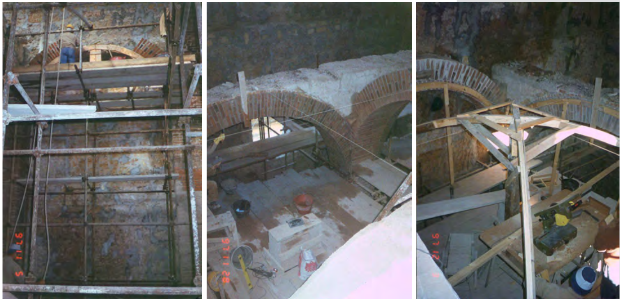
Figures 14, 15, 16. Construction of perimeter arches, using solid bricks and supporting the timbered vaults.
