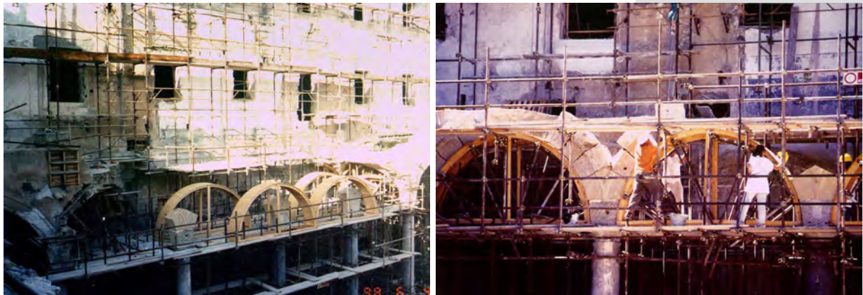
Figures 6, 7. Realization of wooden supporting structure of stony arches and of the carved stony ashlars of portico arches.
