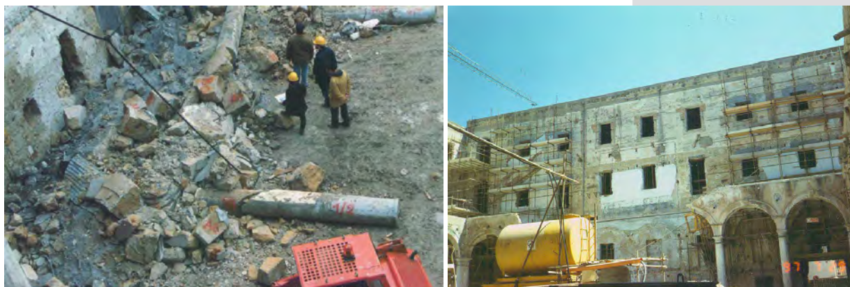
Figures 1, 2. Collapse following a mafia-style vandalism and related survey construction phases.
