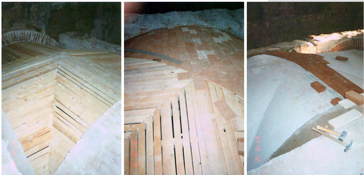
Figures 17, 18, 19. First "sheet" of thin dry bricks and second sheet of bricks overposed on the still fresh layer of gypsum paste.
