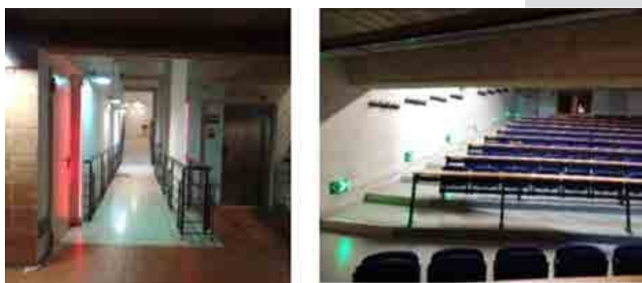
Figure 6. CBE application in the building: along the corridors, the evacuation path was addressed by LED stripes portals placed on the wall (left), to address usable paths (green lights) and prohibited paths (red lights); in the classroom, the evacuation direction was addressed by directional (LED) arrows, placed on the wall, straight to the floor level (right).
