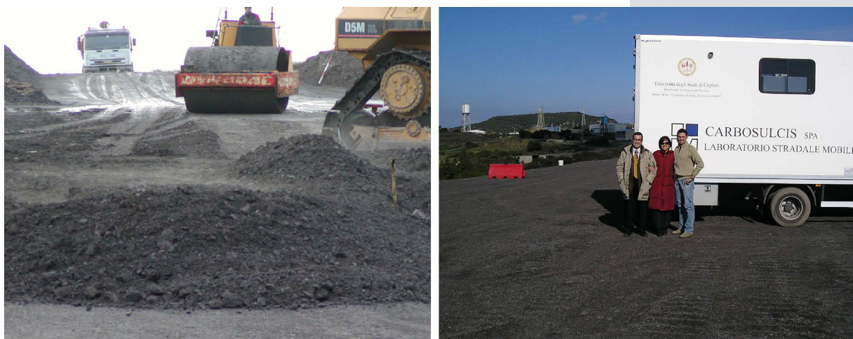
Figure 2. The road embankment built in 2007 with the coal waste inside the Carbosulcis mining site.
