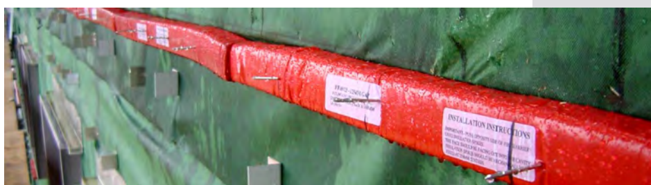
Figure 7. Example of fire barrier used to limit the fire spread in a ventilated layer (Tenmat Fire barriers, BBS Facades Ltd).
