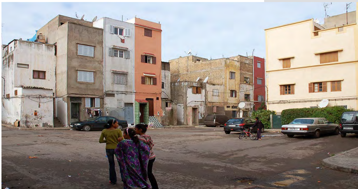
Figure 3. The mutation of the houses of the “Omer” type has not altered the structure of the public space originally foreseen by the Azagury project (photo by S. Mocci).
