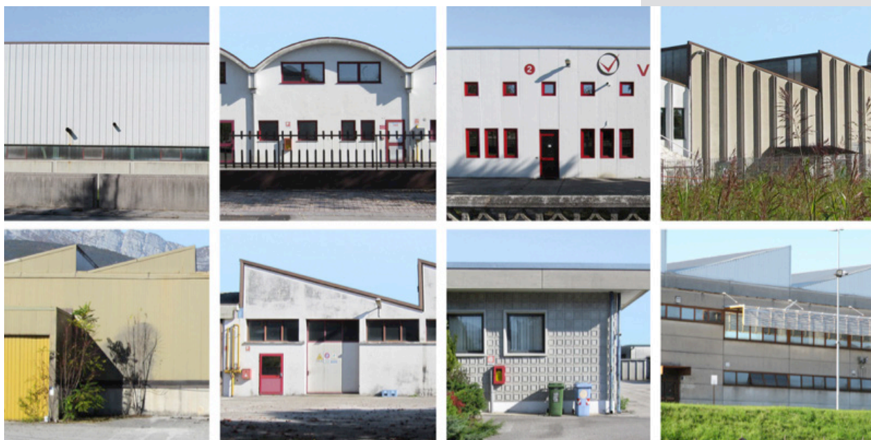
Figure 1. Industrial buildings in the district in Maniago (PN): types of building, building systems and materials: reinforced concrete structures and sandwich panels, reinforced concrete structures and masonry in brick or concrete blocks, precast concrete structures and panels.
