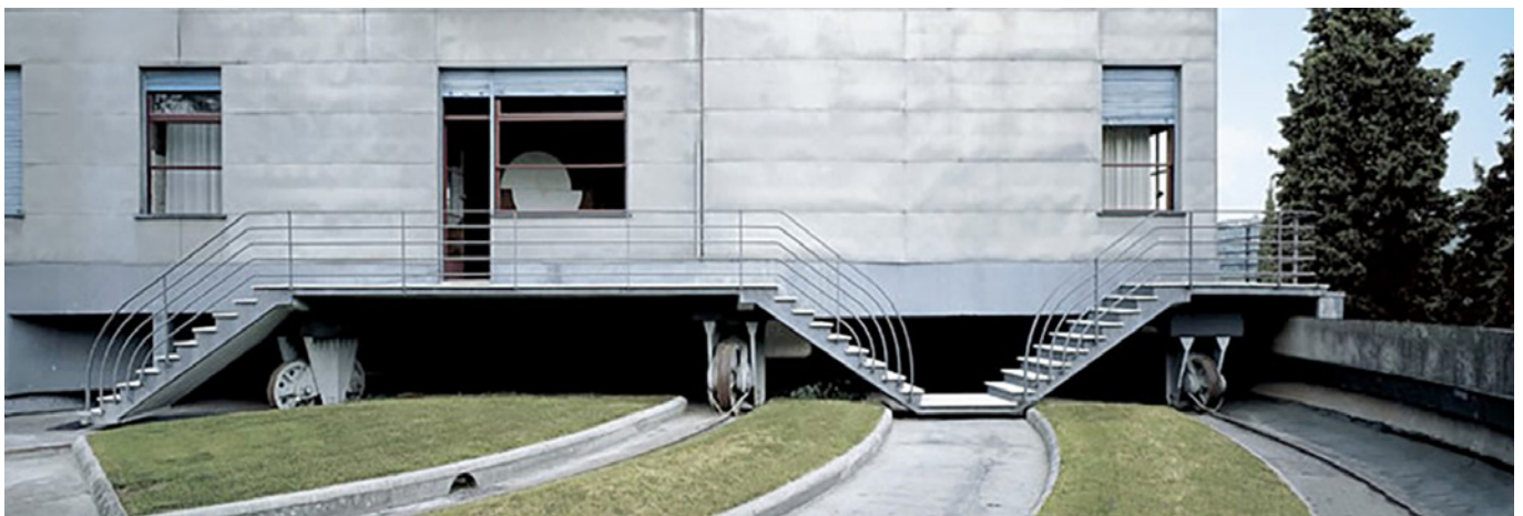
Fig. 8. Coating of the external surface with Alumàn slabs, produced by the company "Lavorazioni Leghe Leggere" (Image source: FAI – Fondo Ambiente Italiano).
