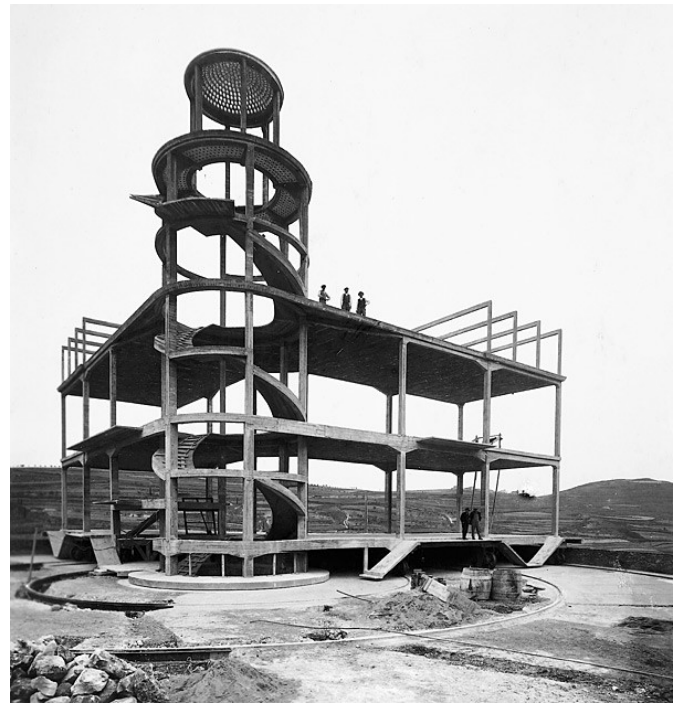
Fig. 7. Reinforced concrete structure of Villa Girasole. (Image source: Galfetti A, Frampton K, Farinati V, 2016).
