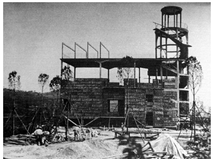
Fig. 10. The external wall built in “Eraclit” blocks (Image source: Galfetti A, Frampton K, Farinati V, 2006).
