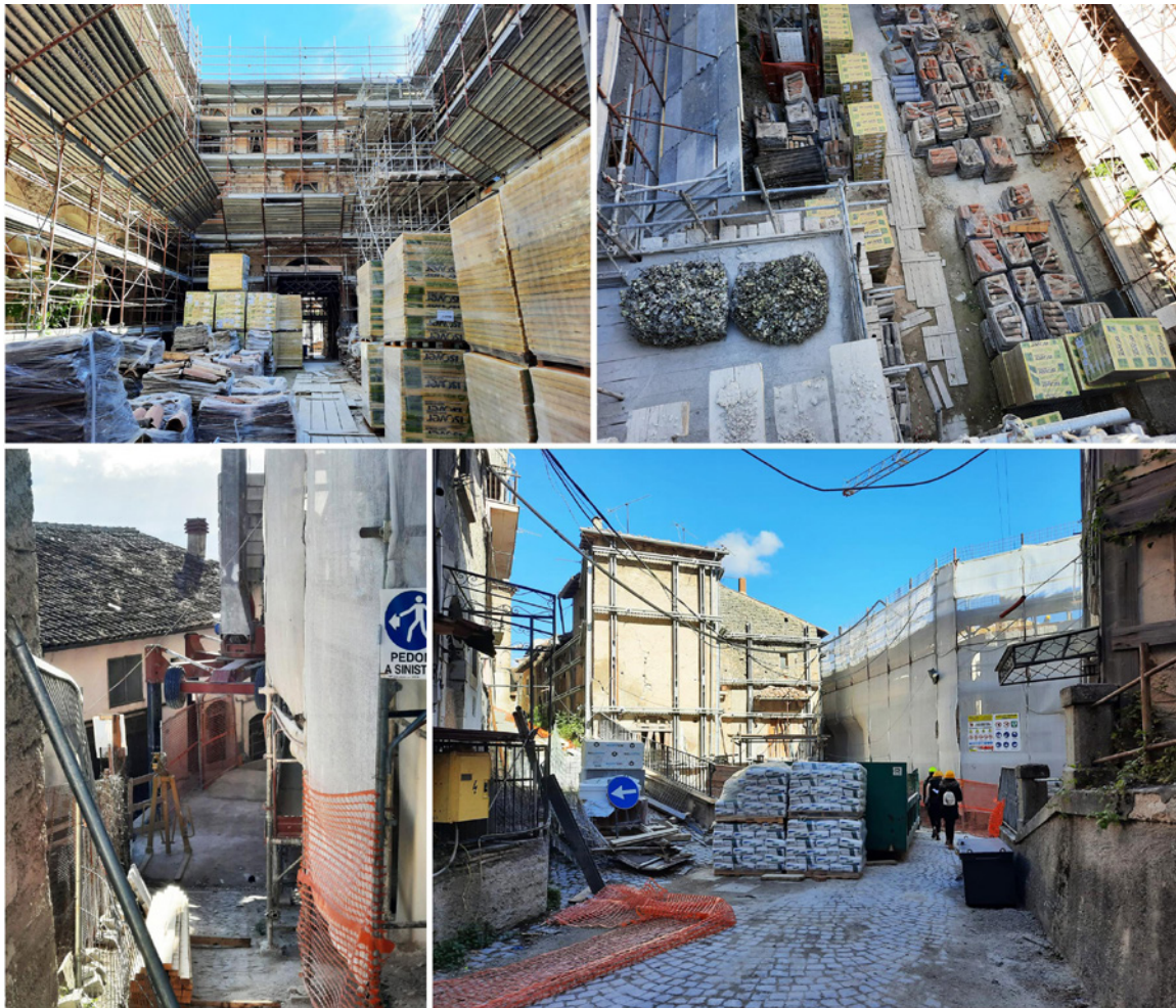
Fig. 1. Logistics criticalities in a built heritage recovery site. Top: Storage areas located in internal courtyards or on scaffolding due to limited availability of space (Construction site after the 2009 earthquake of the E. De Amicis school – L'Aquila). Down: Auxiliary factors management in post-earthquake reconstruction (Fossa, AQ), such as installing cranes using telescopic legs or material storage tailored to reduce interferences with public pedestrian walkways.
