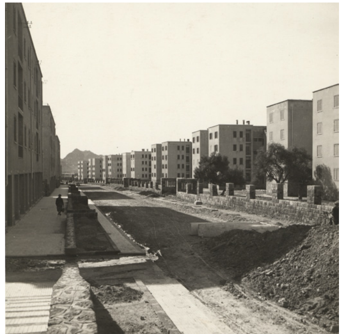
Fig. 8. The Pistoni along Corso Iglesias built with trachyte masonry and brick vaults in an area south of Rio Cannas. In both cases, the works were carried out by the Pasotti Company. (Image source: MAXXI Archive).
