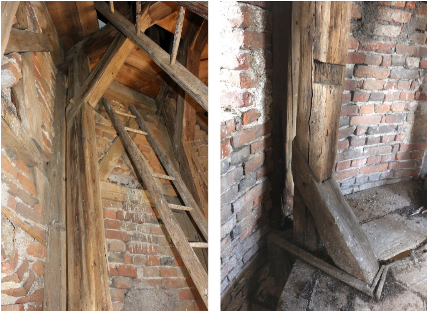
Fig. 5. Clock Tower, half-timbered construction, the traces of the older timber construction. (Photo, 2020).
