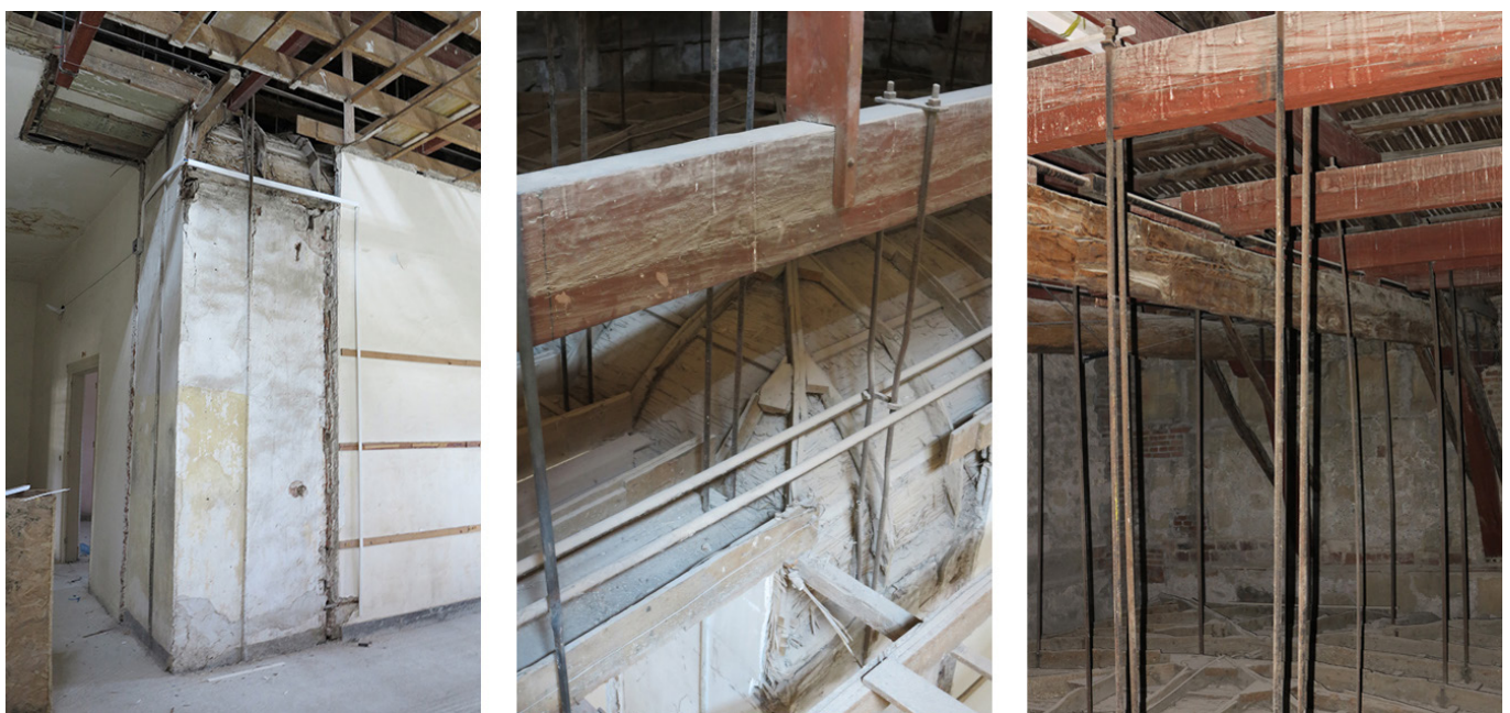
Fig. 5. Thin-tile brick partitions and corresponding timber vaulted ceiling. Some iron tie rods are visible on the surface of the lightweight wall.
