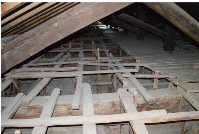
Fig. 10. Ceiling without upper wooden deck with non-uniform arrangement of joists (Rome, Sant’Agnese fuori le mura, extrados of the coffered ceiling, 1606).
