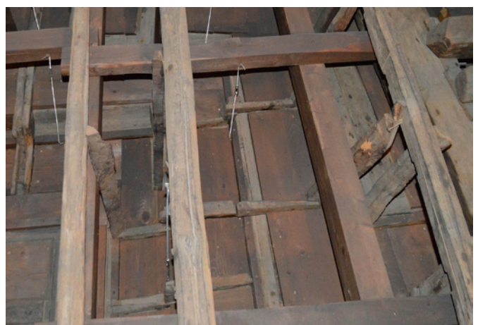
Fig. 7. U frame with a crosspiece made up of several elements connected to each other in a staggered form. The picture shows the reinforcement work carried out about ten years ago, proving the insertion of a little reinforcing steel with double screw clamps for the anchorage of the bottom. In fact, the ceiling presented a marked transversal viscous deformation accompanied by localized subsidence (Rome, San Silvestro al Quirinale, 1573).
