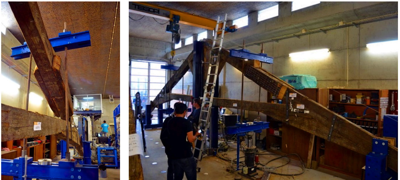
Fig. 5. Repair of a timber rafter using large pieces of wood screwed at the sides of the rafter [14].
