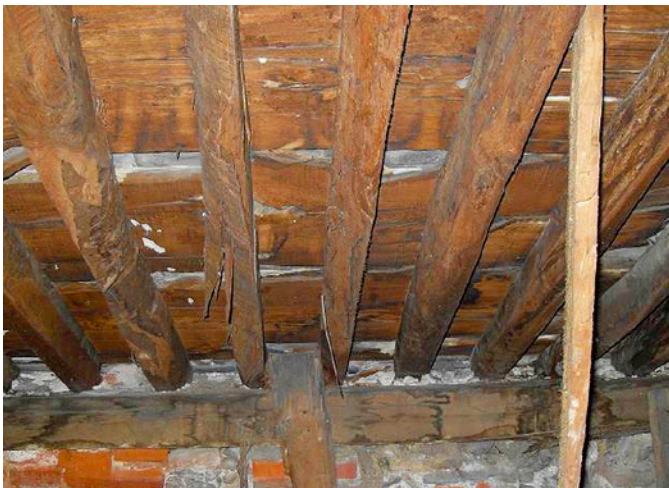
Fig. 9. Cracks and rotting of the rafters.
