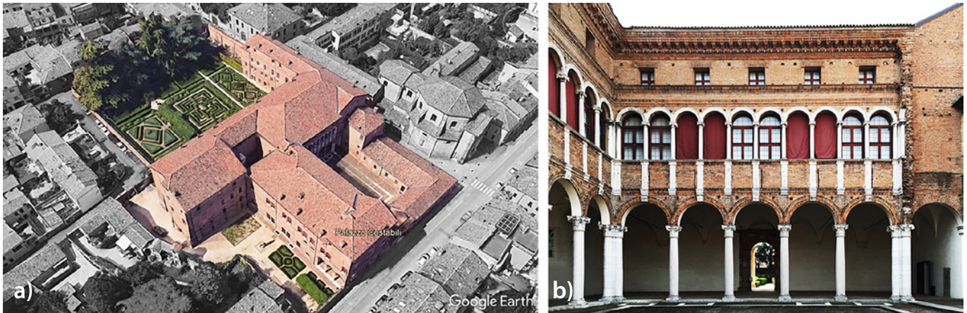
Fig. 1. (a) Aerial view of Palazzo Costabili (image source: Google Earth); (b) three-story building with double loggia organized around the main courtyard.
