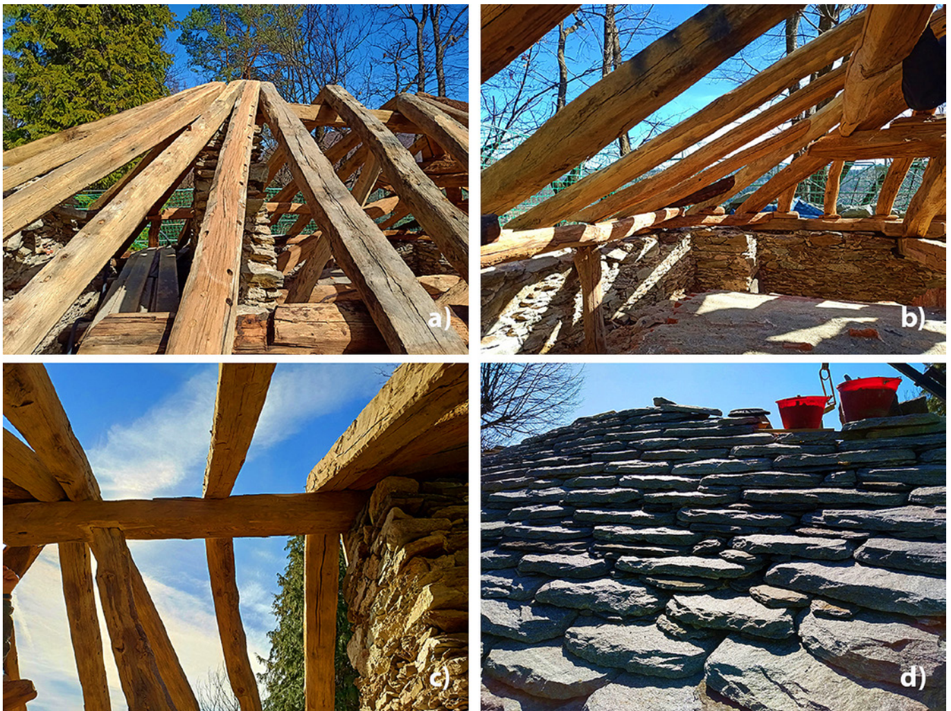
Fig. 10. (a) Placement of new timber elements alongside the original ones cleaned up; (b) integration of the new quay beams into the original structural scheme; (c) cleaning and static improvement of the area around the ridge beam; (d) reconstruction of the original stone roof covering.
