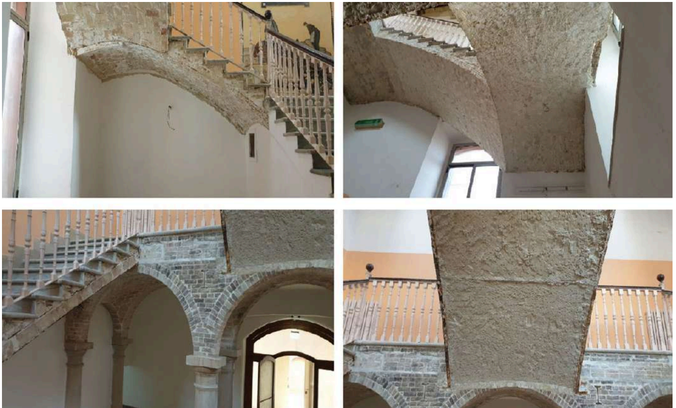
Fig. 7. Construction details: transversal flight from the ground to the first floor (top left); flights ending on the second floor (top right); flights showing metal edge beams (bottom left) and connecting tie rods (bottom right).
