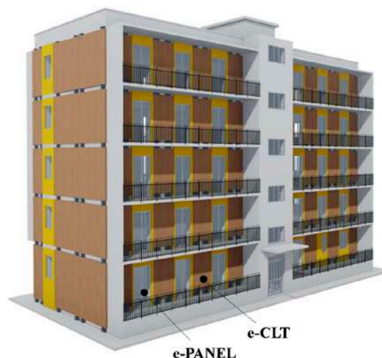
Fig. 7. Pilot building in its current state (a); application of e-PANELS and e-CLTs to the pilot building (b).
