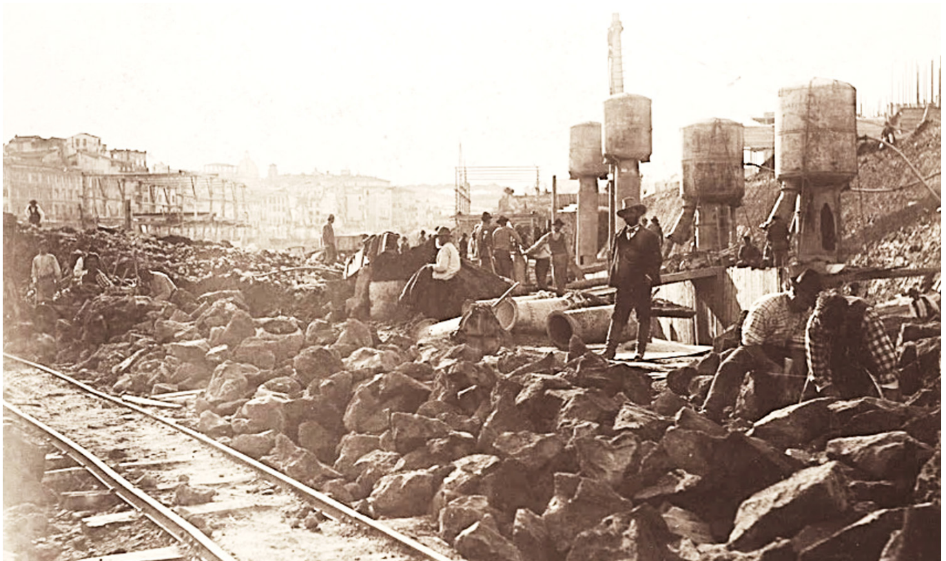
Fig. 7. Pneumatic foundations works on the Tiber's banks, picture by G. Primoli, 1888-90 (courtesy of Fondazione Primoli).
