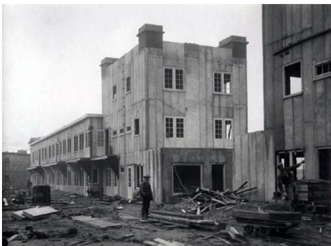
Fig. 4. Quartiere Betondorp (1921-1930), view of the construction site of a building made with «B.B.B. - Bims Beton Bouw» (left) e «Hunkemüller» (right).
