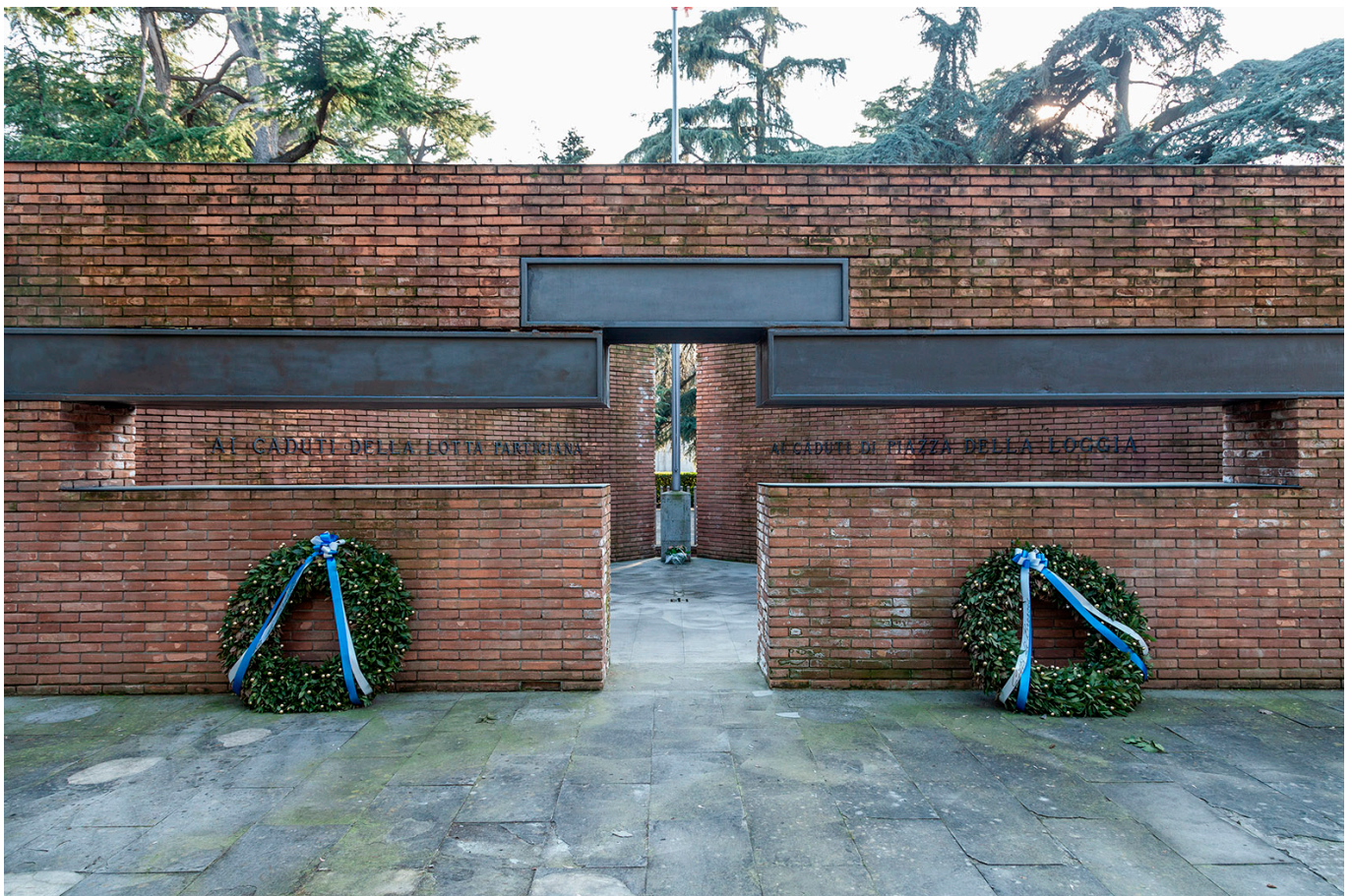
Fig. 3. Gardella's Monument, north façade, 2023.
