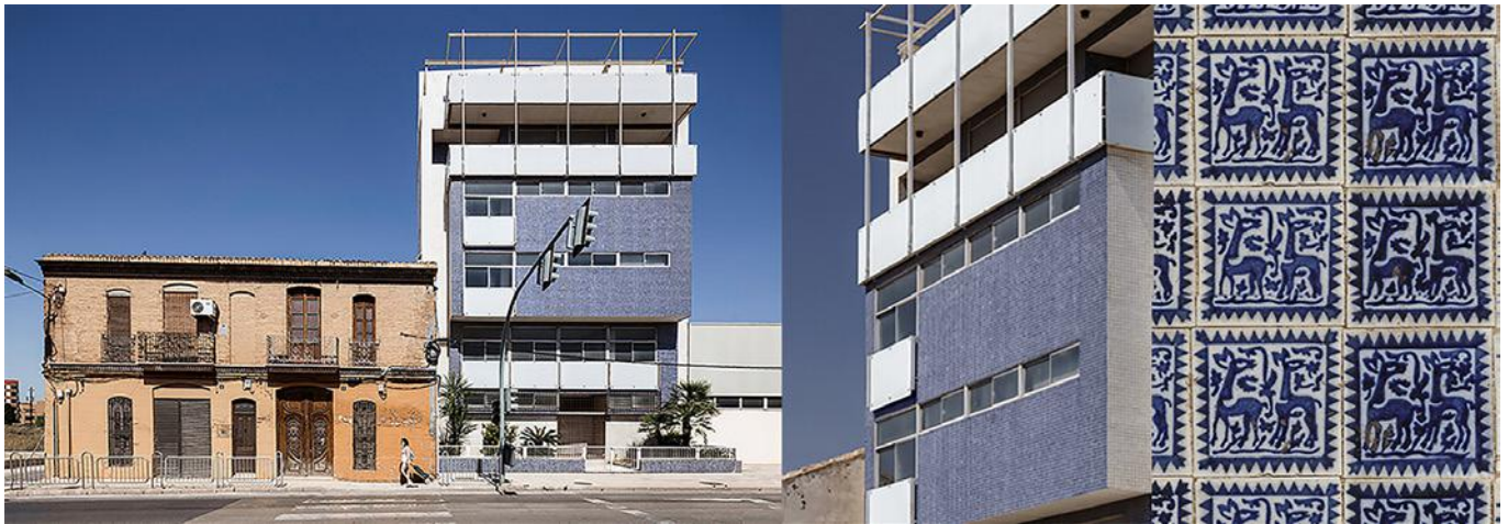
Fig. 8. Rafael Tamarit Pitarch, Enrique Hervás, Hermanos Lladró Building, 1965. Source: © Historical Archive of the Territorial College of Architects of Valencia. Legacy Rafael Tamarit Pitarch. Pictures by Alejandro Gómez Vives.
