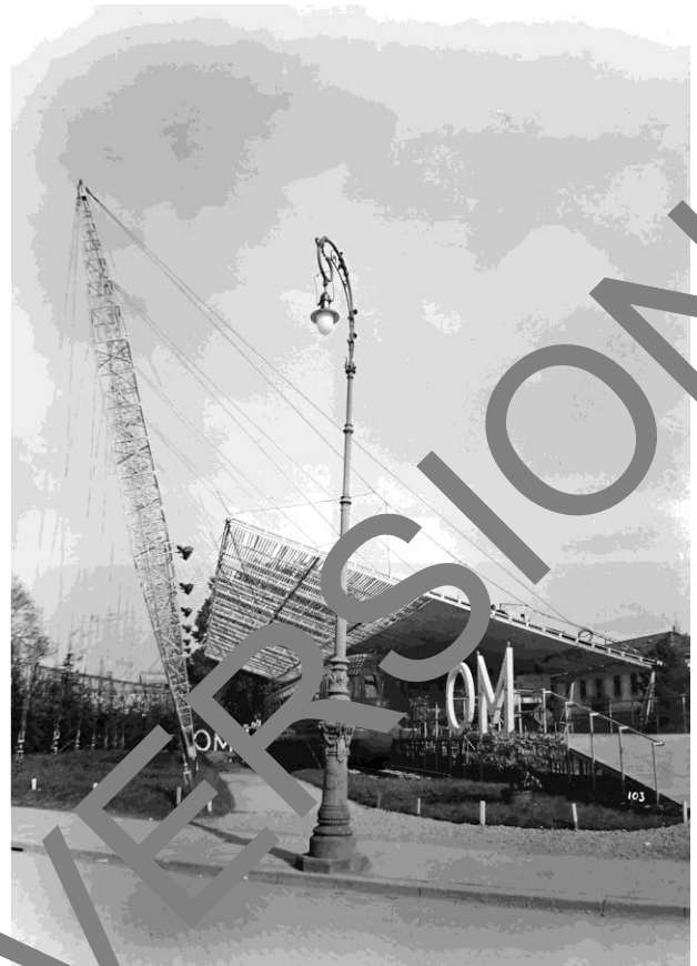
Fig. 2. The OM shelter at the Fiera Campionaria of Milan, 1950: the canopy under construction (left) and the realized building with the suspended cable roof (right). Source: Centro Studi e Archivio della Comunicazione, Università degli Studi di Ferrara - Renzo Zavarella Collection.
