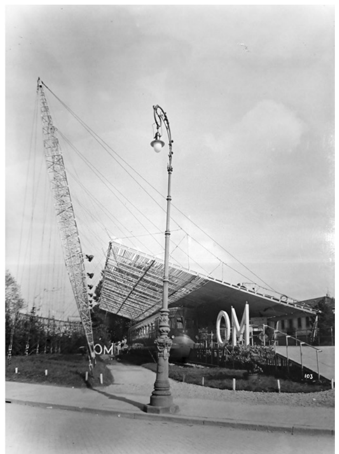
Fig. 2. The OM shelter at the Fiera Campionaria of Milan, 1950: the canopy under construction (left) and the realized building with the suspended cable roof (right). Source: CSAC, Università di Parma, Renzo Zavarella Collection.
