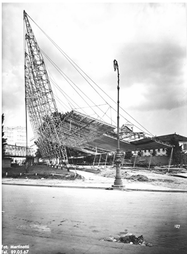
Fig. 2. The OM shelter at the Fiera Campionaria of Milan, 1950: the canopy under construction (left) and the realized building with the suspended cable roof (right). Source: CSAC, Università di Parma, Renzo Zavarella Collection.
