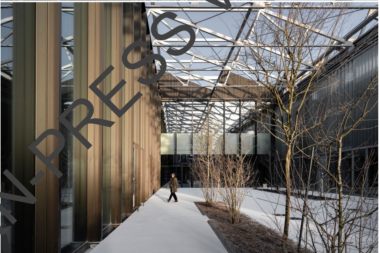
Figure 5 - The façade on Via Tortona treated as a continuous shop window and the internal courtyard with the permeable roof built of steel trusses (© Andrea Martiradonna).
