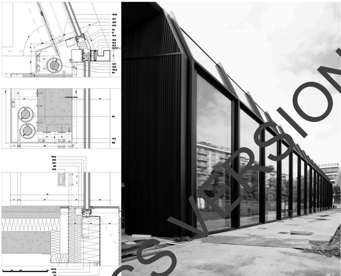
Figure 4 - The transparent facade on Via Tortona with the upper part shaped as the backward roof of the previous industrial building (© Park Associati).
