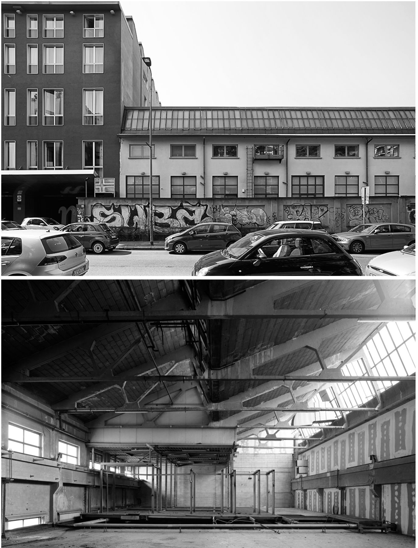
Fig. 2. The façade along Via Tortona and the interior space of the GE factory placed next to the building block redesigned by Alfredo Beretta and Matteo Thun. Source: © Park Associati.
