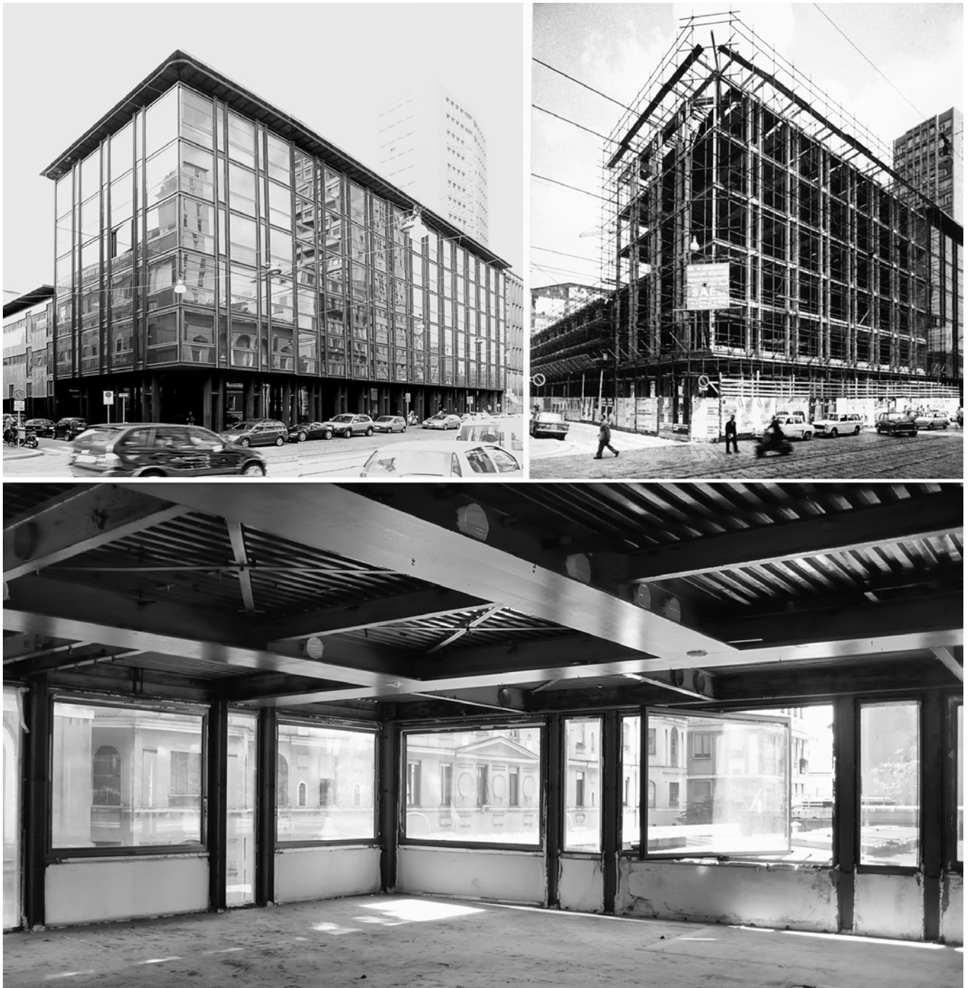
Fig. 6. The original office building La Serenissima placed on Via Turati and designed by Ermenegildo and Eugenio Soncini . Sources: © Park Associati ; Archivio Soncini – © Comune di Milano – CASVA ; © General Planning .
