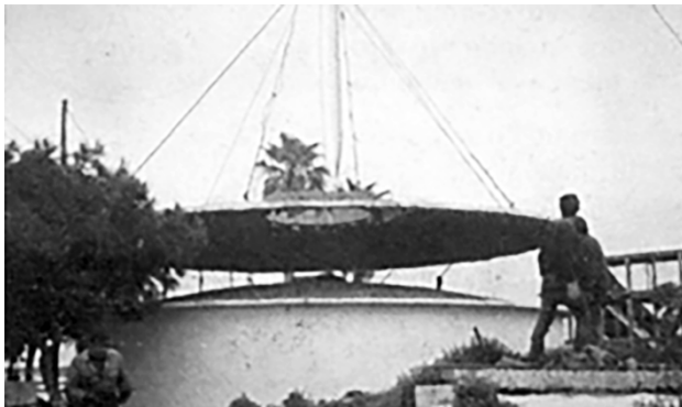
258 Fig. 5. Top left: Transportation of two of the arsenal vaults. Top right: Structural section showing vault reinforcing bars and steel 259 reinforced mesh. Bottom left: Lifting the dome from the tank used as formwork. Bottom right: Structural section of the dome. Images 260 by Kalemkerian et al., 1976.
