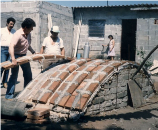
Fig. 4. Left: Carlos González Lobo raises a costilla from the mold. Right: Connections of the costillas with the main structure. Images by Gonzalez Ortiz, 2001.
