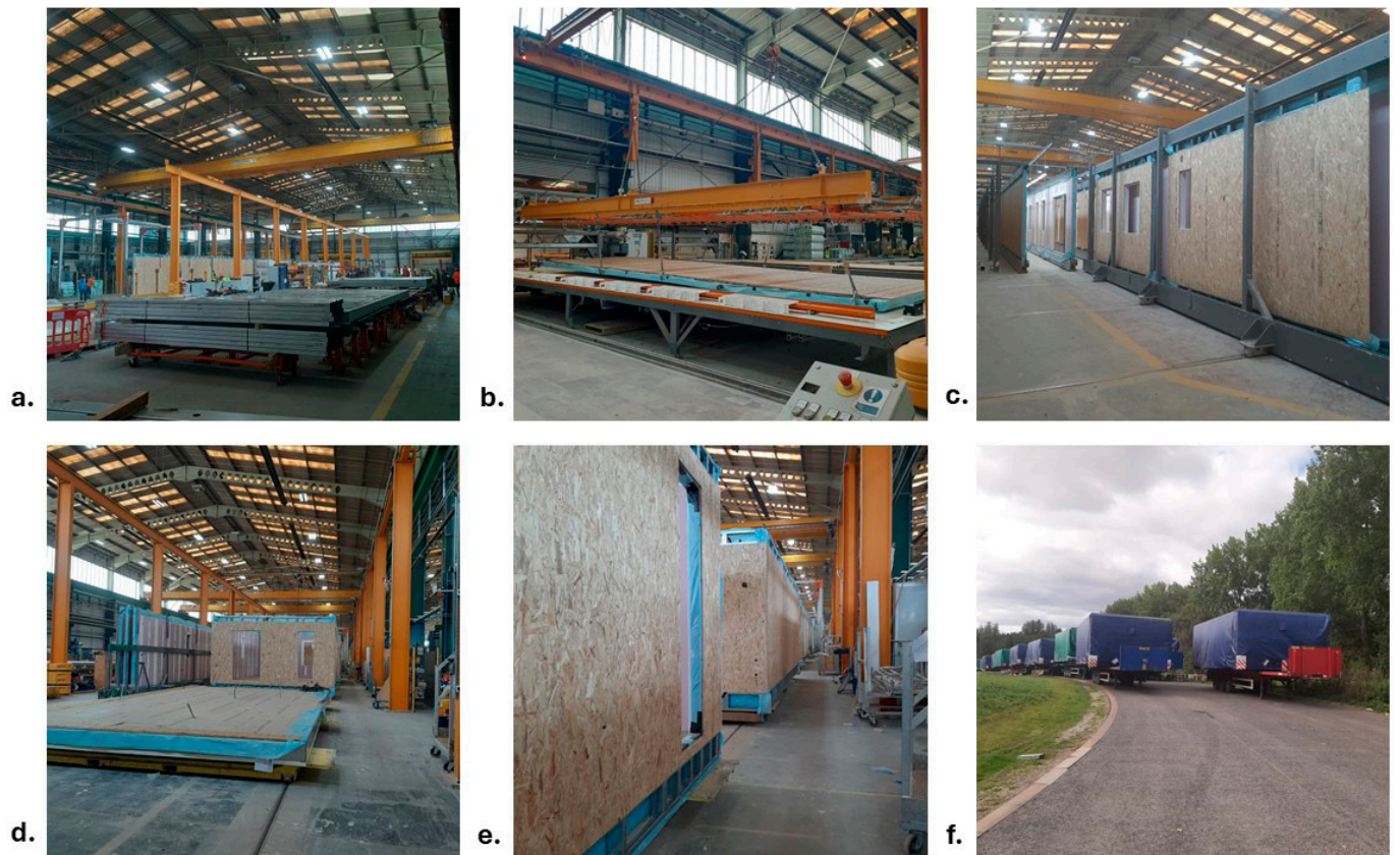
Fig. 6. Production line of the developed modular system showing: (a) ground floor assembly; (b) high-speed panelizing system for connecting the sheathing boards to the wall steel frame; (c) line production of the walls; (d) assemblage of the floor and wall system; (e) line production of the volumetric modules; (f) modules ready to be transported on-site for assembly.
