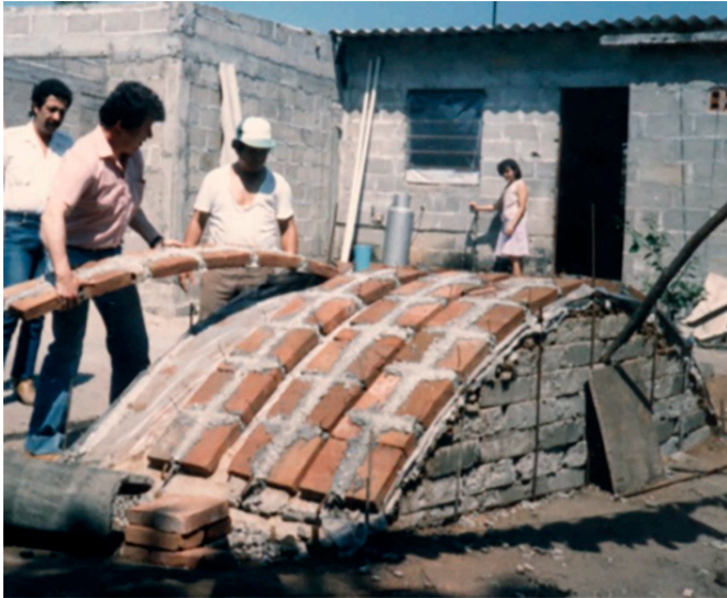
Fig. 4. Left: Carlos González Lobo raises a costilla from the mold. Right: connections of the costillas with the main structure. Source: [26].
