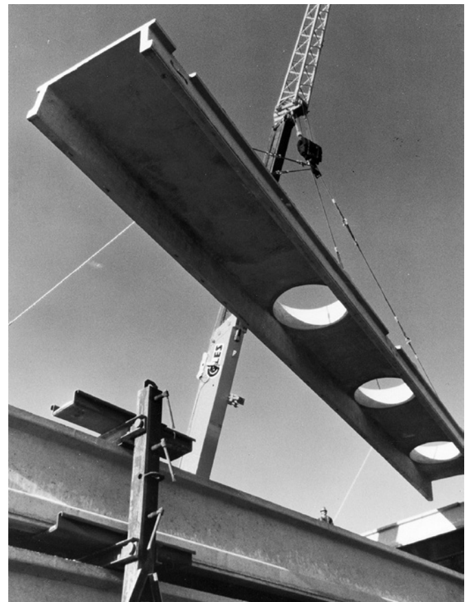
Fig. 9. IBM Italia factory, view of the building site during assembly of the U-shaped roof tiles. Source: Archivio del Moderno, Fondo Marco Zanuso, Balerna.
