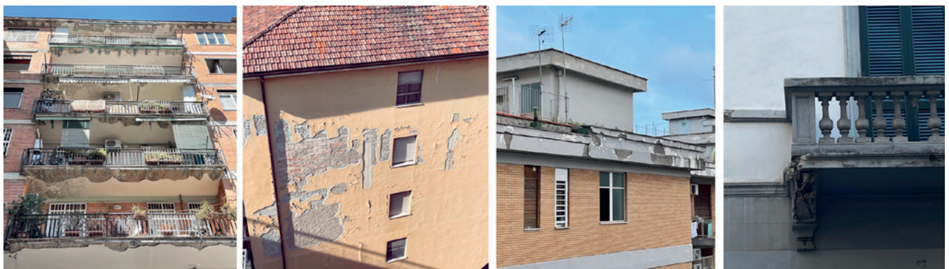
Fig. 1. Examples of damaged cornices, balconies, plasters, and decorations.
