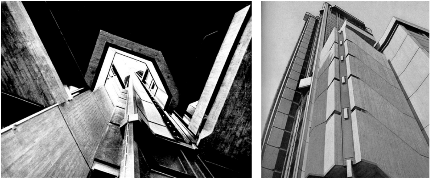
Fig. 9. The load-bearing corner elements breaking through the base and cellular concrete panels of the distribution area. Source: © Archivio Edilizia Privata, Comune di Genova.
