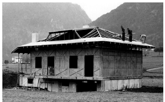
Fig. 8. From the top, the assembly of a house with "Block-Volume" produced in the factory and plastered on site in the first years after the 1976 earthquake. Source: © E.M.E. Ursella Srl, 2024.
