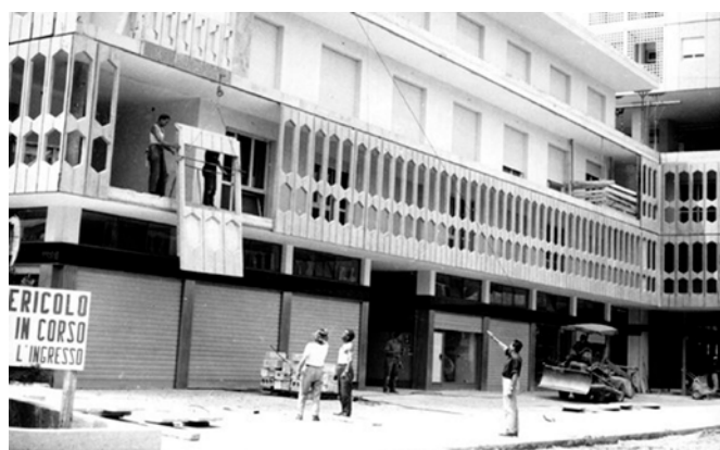
Fig. 6. Top: Lignano City with Palazzo Celeste and Palazzo Rosato. Bottom: site phases of the assembly of the perimeter closure panels of Palazzo Celeste in Lignano City. Source © E.M.E. Ursella Srl, 2024.
