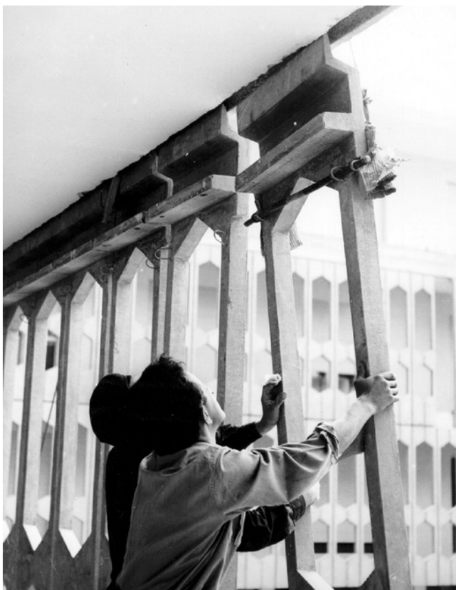
Fig. 6. Top: Lignano City with Palazzo Celeste and Palazzo Rosato. Bottom: site phases of the assembly of the perimeter closure panels of Palazzo Celeste in Lignano City. Source © E.M.E. Ursella Srl, 2024.
