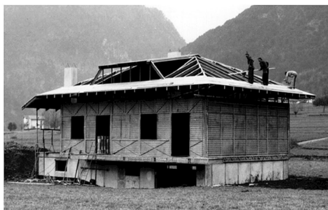
Fig. 8. From the top, the assembly of a house with "Block-Volume" produced in the factory and plastered on site in the first years after the 1976 earthquake. Source: © E.M.E. Ursella Srl, 2024.
