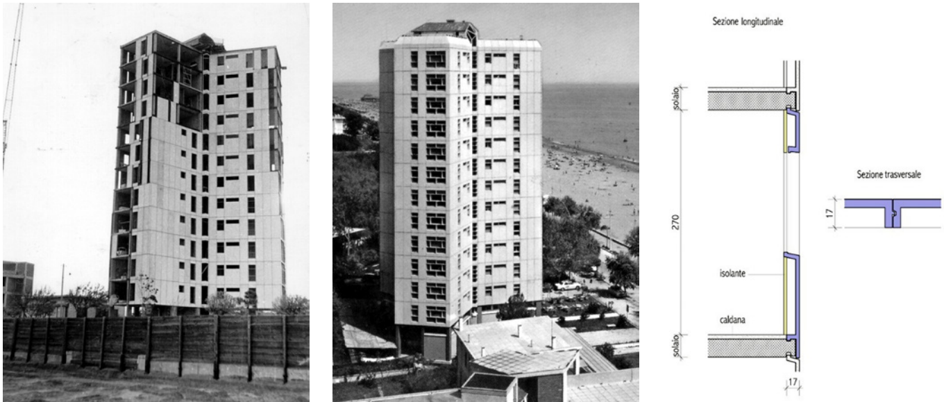
Fig. 5. Torre di Zainer in Lignano Sabbiadoro. Left: the site assembly phase. Middle: the final realisation. Source: © E.M.E. Ursella Srl, 2024. Right: detail of the lower groove of the slab, with particular reference to the lower and upper splines and the “male-female” joint in the cross-section. Source: [12].
