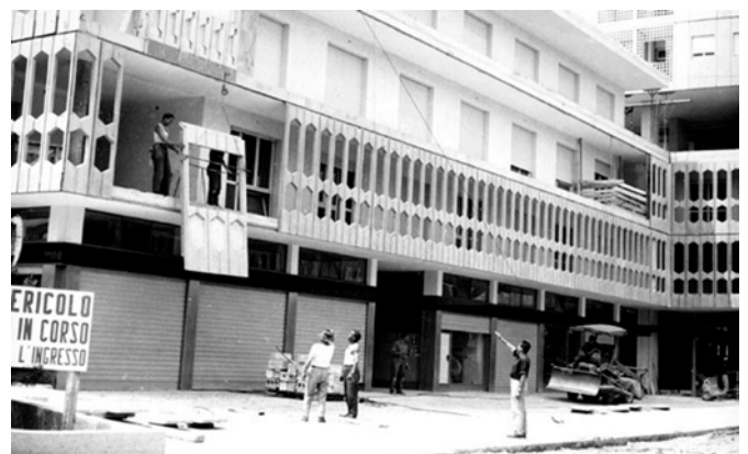
Fig. 6. Top: Lignano City with Palazzo Celeste and Palazzo Rosato. Bottom: site phases of the assembly of the perimeter closure panels of Palazzo Celeste in Lignano City. Source © E.M.E. Ursella Srl, 2024.
