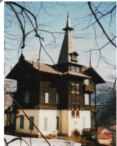
Figs.7, 8: Villa Piaggio researches. The villa was designed by R. Haupt in 1907. The load-bearing structure on the ground floor has exposed timber pillars and rafters. On the upper floor, there is a timber cladding with industrially processed elements. (source: Maraldi's archive)
