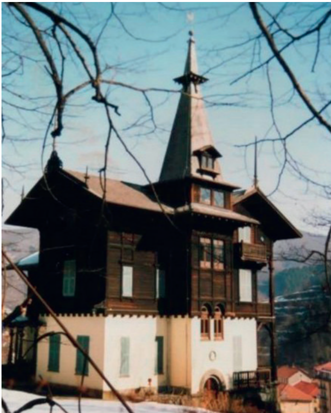
Fig. 8. The load-bearing structure on the ground floor has exposed timber pillars and rafters. On the upper floor, there is a timber cladding with industrially processed elements. Source: Maraldi's archive.
