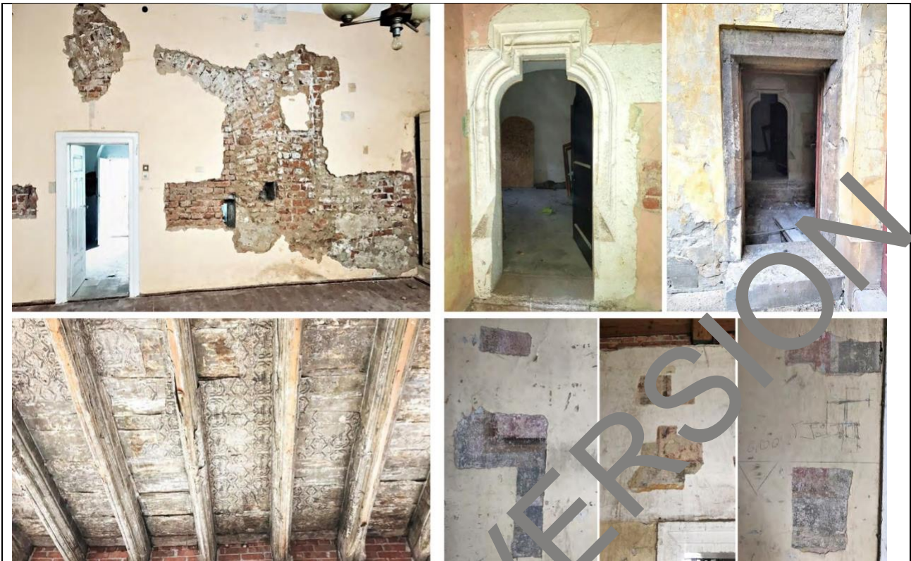
Figure 2 – Images from April 2024: decorative elements and deterioration conditions of the building. From top clockwise: test for masonry stratigraphy; stone portals on the ground floor for access to the original chambers, wooden ceiling with tapestry typical of Krakow buildings of time, sample for masonry decorations. CC-BY ©2025, J.S.
