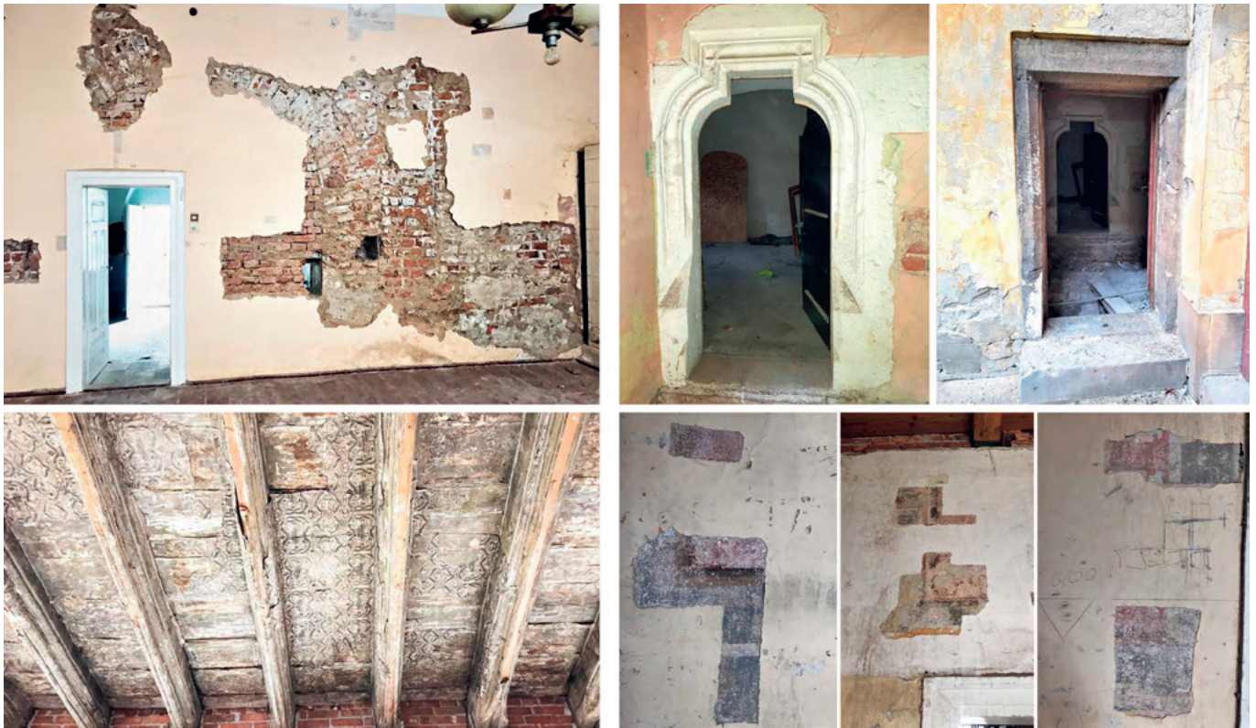
Fig. 2. Images from April 2024: decorative elements and deterioration conditions of the building. From top clockwise: test for masonry stratigraphy; stone portals on the ground floor for access to the original chambers, wooden ceiling with tapestry typical of Kraków buildings of time, sample for masonry decorations. Source: CC-BY; © 2025, J. S.
