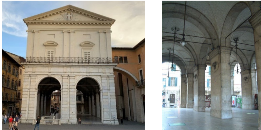
Figure 1 – “Logge di Banchi” in Pisa. Façade view and internal view of the loggia.
